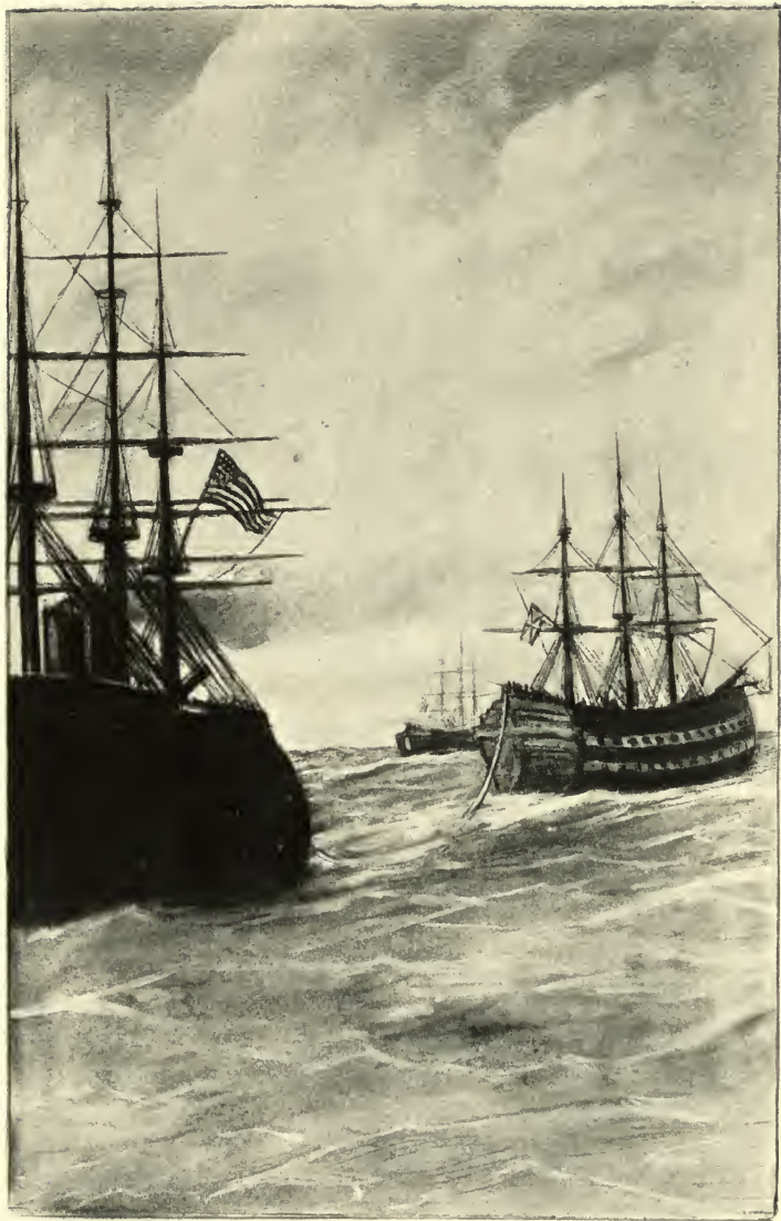
There, midway between the nations, they spliced the cable.
